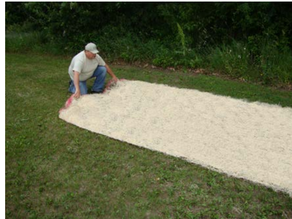
Figure 4. Properly position unrolled RECP for installation.
