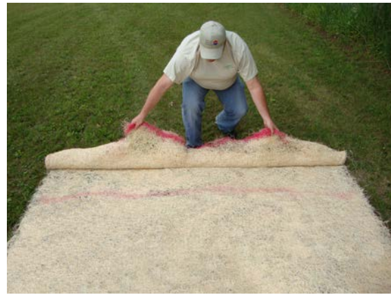
Figure 2. Pull end of RECP along red dye line.
